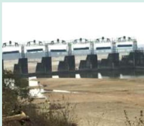
Infrastructure (Barrage) to divert water from the river to the irrigation canals
