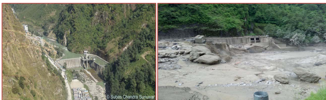
Upper Bhotekoshi HEP Headworks before Flood and After Flood (Pic. Mr.Subas Chandra Sunuwar and Er. Kapil Dhital respectively)
